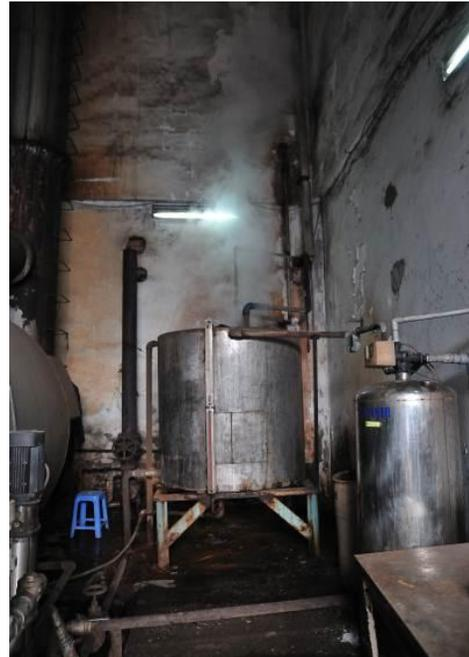
*Open and no-insulation tank of condensed water*
